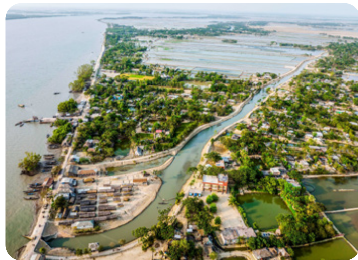
Mangrove clearance in Satkhira, Gabura, Bangladesh, adjacent to the Sundarbans. © FAO-GMB Akash.
